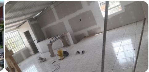
Tile on 2 nd Floor nearing finish
