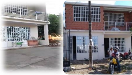
Progress of FRONT LAMB Ministries HQ
